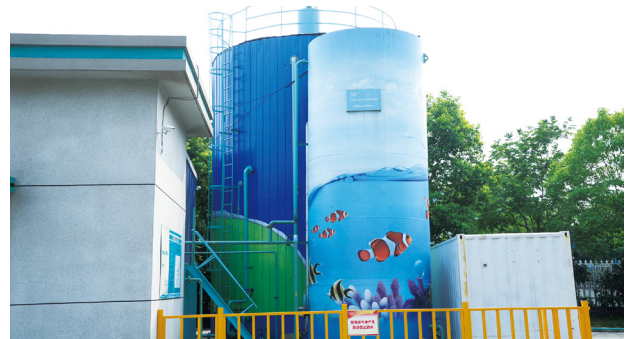
Anaerobic Tower for Sewage Treatment in Huzhou Production Base
